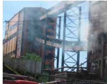
Pict. 6: Fire on conveyor bridges
