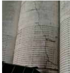
Pict. 4: Silo cell after fire
