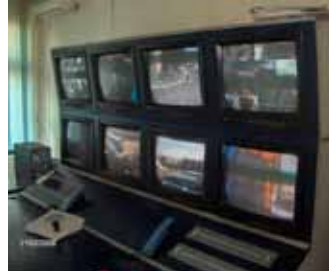
Pict. 14: Control panel of a video surveillance
