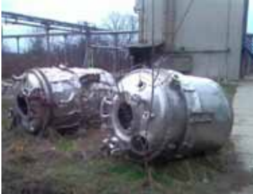
Pict. 9: Vessels after explosion in chemical industry
