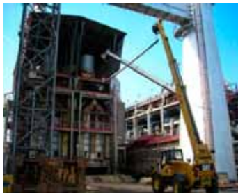
Pict. 11: Oil refinery furnace repair
